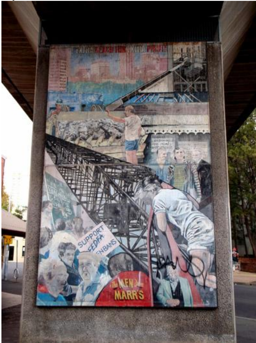
One of the 1981 panels on the Woolloomooloo Viaduct. These panels are now in poor condition.
