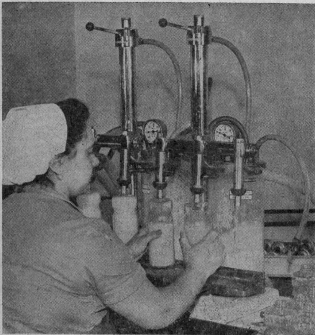
Ready-labelled "Handy Andy" bottles pass swiftly and smoothly through a new filling head operated skilfully by Giama Rando.
