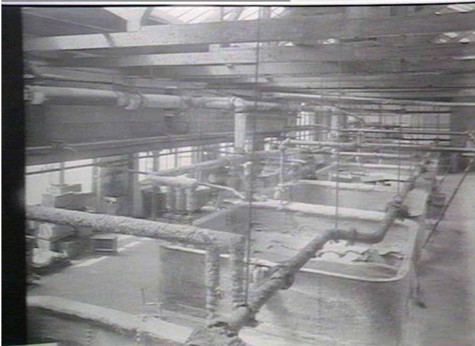
Pan Room where soap was boiled. Lever Brothers, Balmain ca 1935 50 ton capacity soap pans
